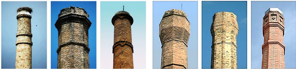
Figure 3: Different types of crowns taken from masonry chimneys in Spain, [14].
