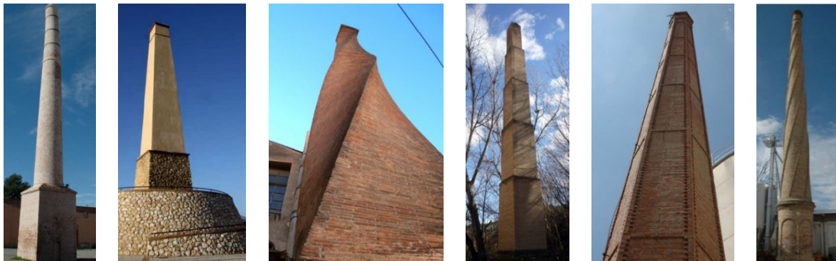
Figure 2: Different examples of chimney's shaft taken from masonry chimneys in Spain, [14].
