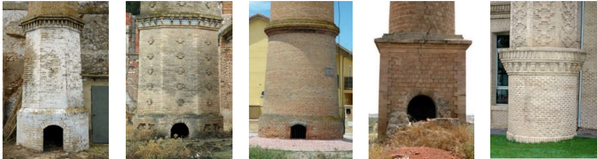
Figure 1: Different configurations of chimney's base taken from masonry chimneys in Spain, [14].
